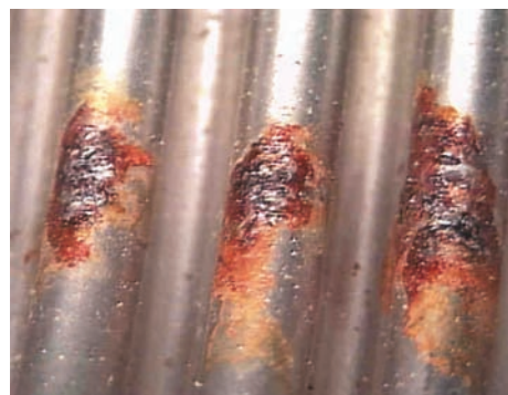
Corrosion form and mechanism Local corrosion, pitting, crevice Material Type 321 stainless steel Product form Convoluted bellows-hose system
