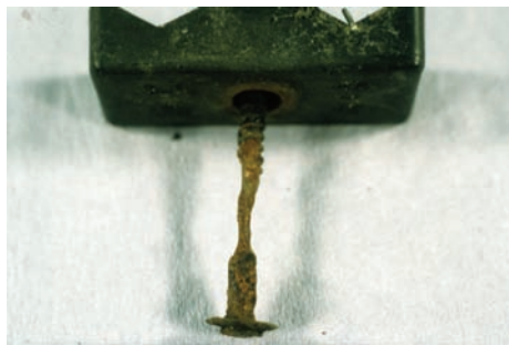
Corrosion form and mechanism Stray-current corrosion, crevice corrosion Material Carbon steel Product form Electric cable support
