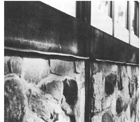
Fig. 14 Use of stiff rubberized sheeting beneath beam to divert drainage beyond stone wall
