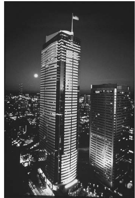
Fig. 10 The Two Union Square building in Seattle, WA, used concrete with a design compressive strength of 131 MPa (19 ksi) in its steel tube and concrete composite columns.
